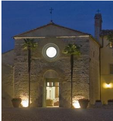
San Fedele - Restored Monastery
